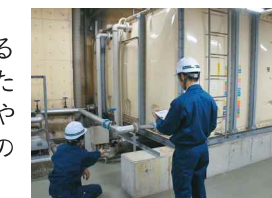
貯水槽の点検
